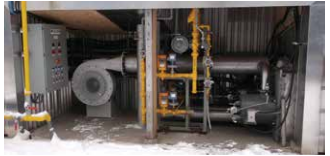
A self contained natural gas heating system that directly drives the steam generator.
